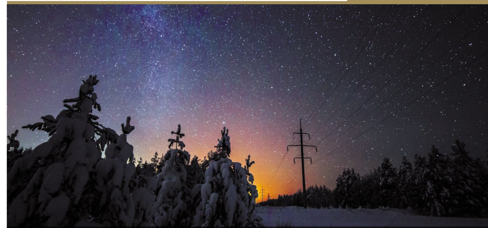
Lighting the Milky Way. Photo by Chalanov Ivan Alexandrovich, category 3 electrician for distribution grids operation at Komienergo branch of PJSC IDGC of the North-West. The photo shows OL-110 kV from SS Ust-Kulom, Ust-Kulom, the Republic of Komi. Winner in the nomination "Nature" of the photo contest "In harmony with nature"
