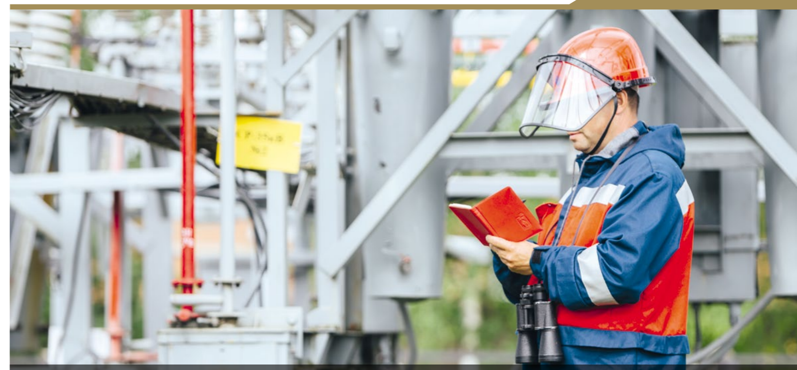
Inspection of the outdoor switchgear at SS 110 kV Lugovaya, Vologdaenergo branch
